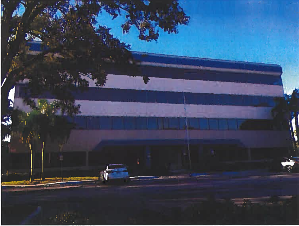
Exhibit A: Main Entrance Facade
