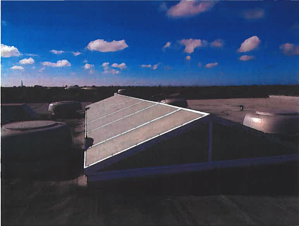
Exhibit G: Roof Skylight
