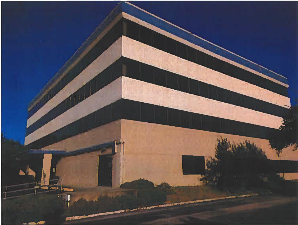
Exhibit B: Precast Concrete and Ribbon Window Facade
