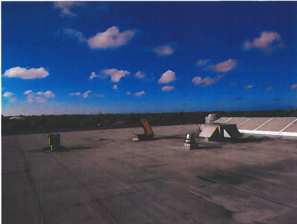
Exhibit F: Roof Field Area with Skylight
